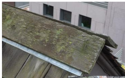
Carriage House ridge cap with mitered, open joint and rusting flashing, November 2014. Photo courtesy of BOLA.
