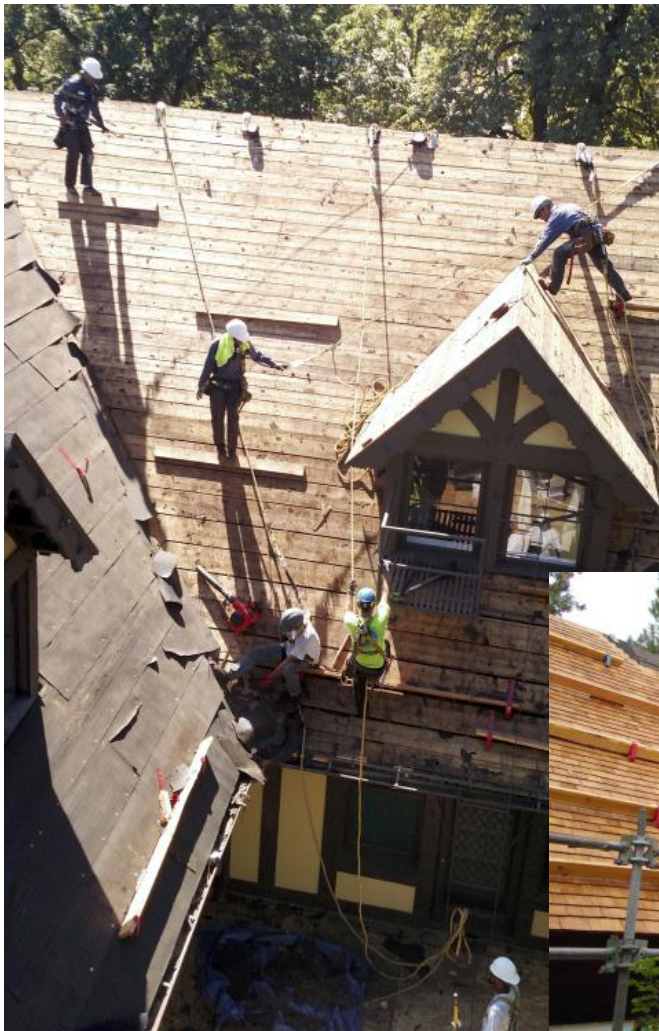
Campbell House during tear-off and sheathing evaluation, showing tight sheathing, August 2016. Photo courtesy of BCI.
