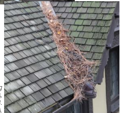
Carriage House ridge cap with mitered, open joint and rusting flashing, November 2014. Photo courtesy of BOLA.
