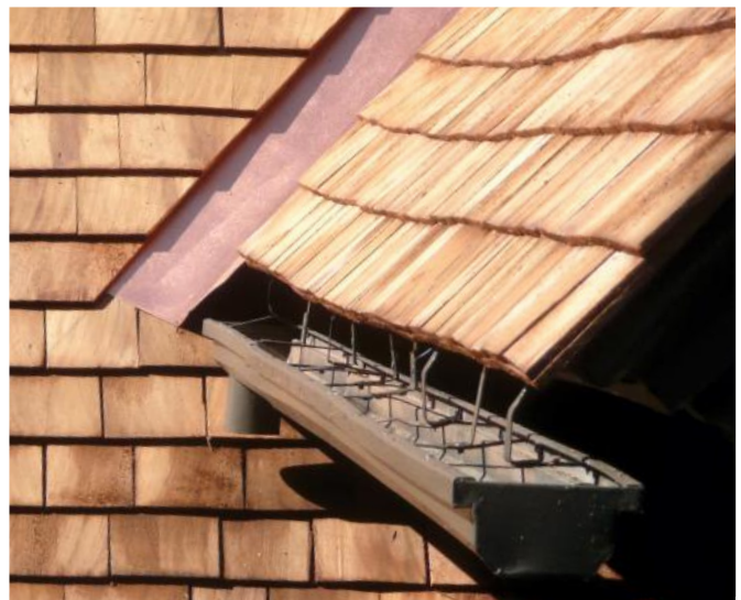
Work included restoring, re-leveling, and re-aligning the drip line of the existing custom shaped and custom hung gutters and downspouts. September 2016. Photo courtesy of BOLA.
