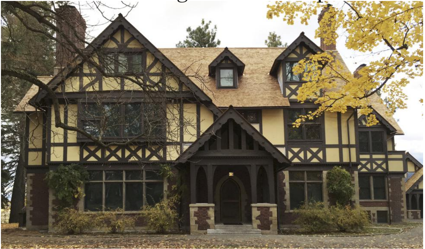
Campbell House Reroof completion, November 2016. Photo courtesy of Northwest Museum of Arts & Culture
