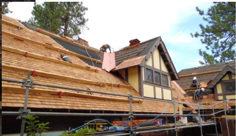
Reroofing the carriage house in 2016. Photo courtesy Tony Hyatt, Cedar Shake and Shingle Bureau.
