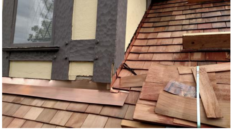
Carriage House dormer, showing step flashing integration with existing base flashing, and adzed trim to be restored, July 2016. Photo courtesy of BCI.
