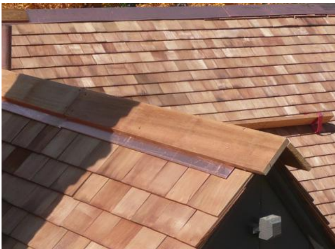
Detail of improved ridge cap. September 2016. Photo courtesy of BOLA.
